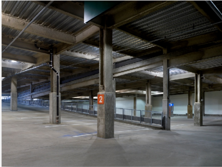
Figure 6: Existing Parking Garage
